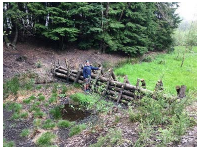
Overland leaky barrier on the upper Pip Brook NFM scheme, Dorking, Surrey (© Jay Neale)
