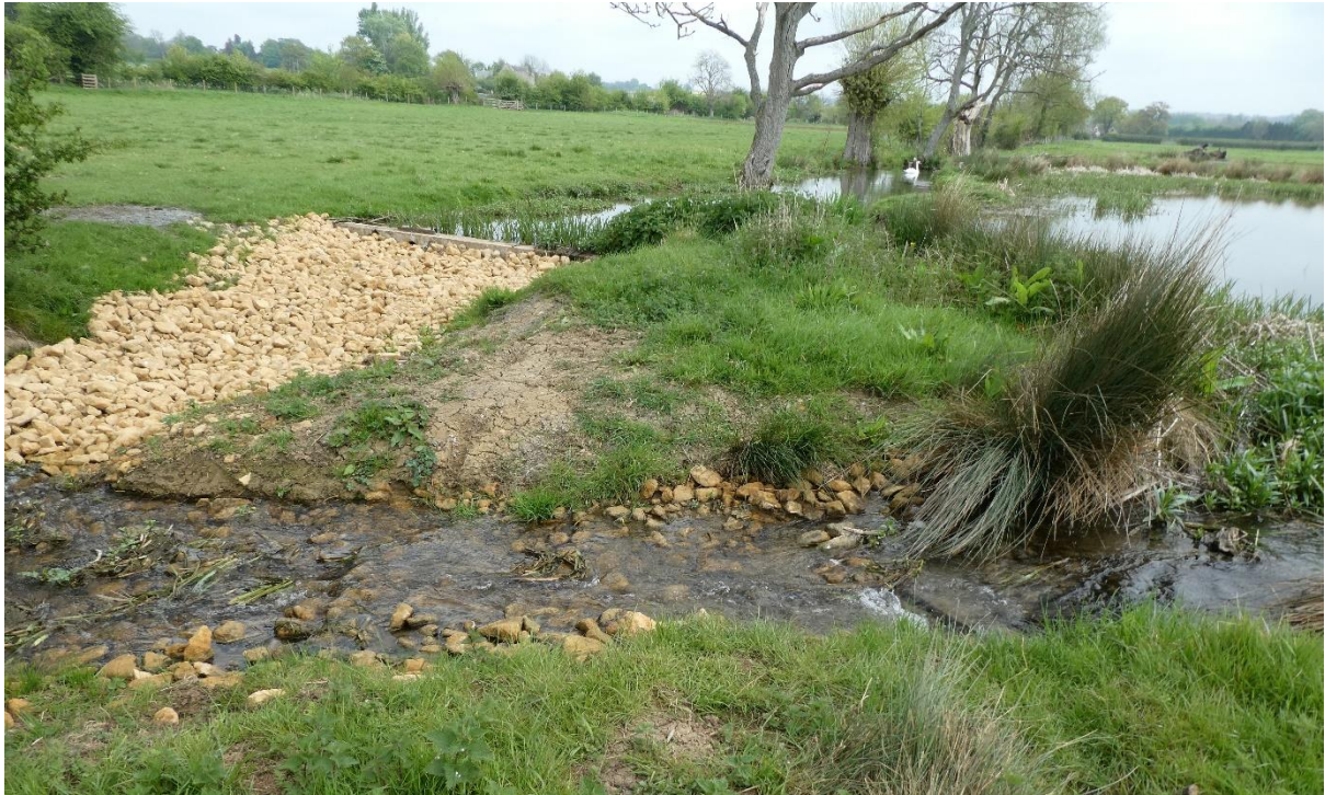
Weir removal, Brookend Farm
