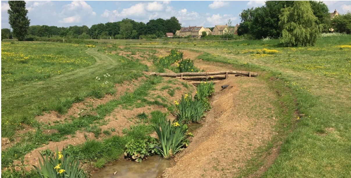
Two stage channel and leaky woody dam at Blenheim Meadow, Moreton in Marsh. @Wild Oxfordshire
