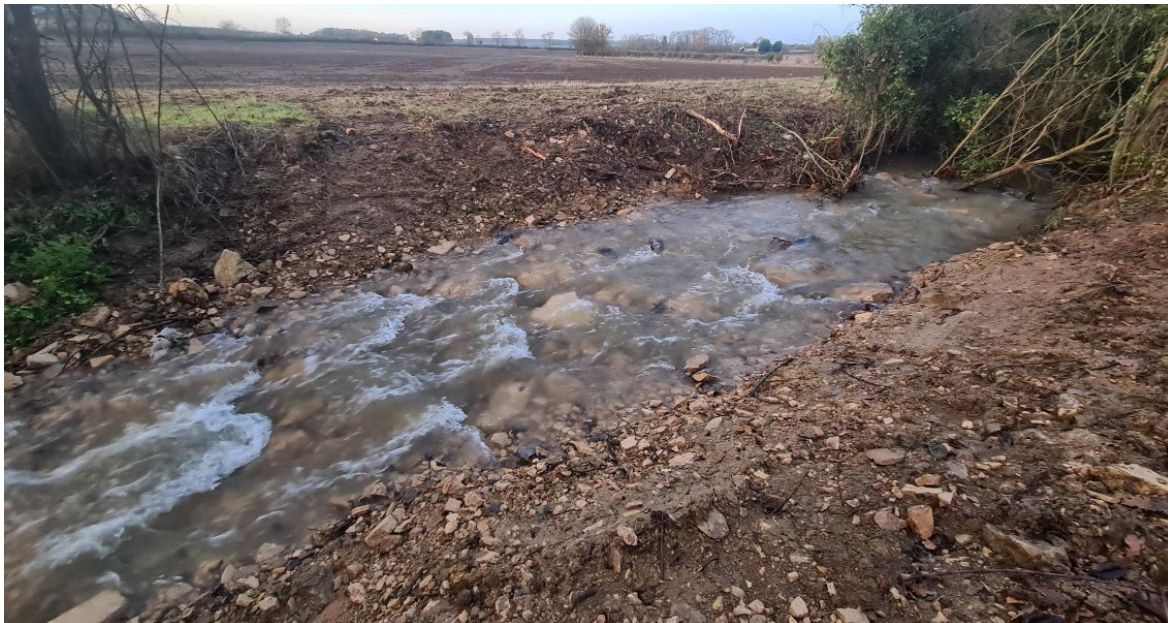
Brook bed restored to continuous gradient. @Wild Oxfordshire
