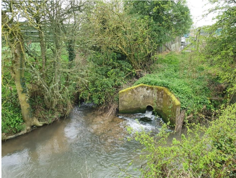
Figure 7-1 The discharge point from MuW STW into Littlestock Brook
