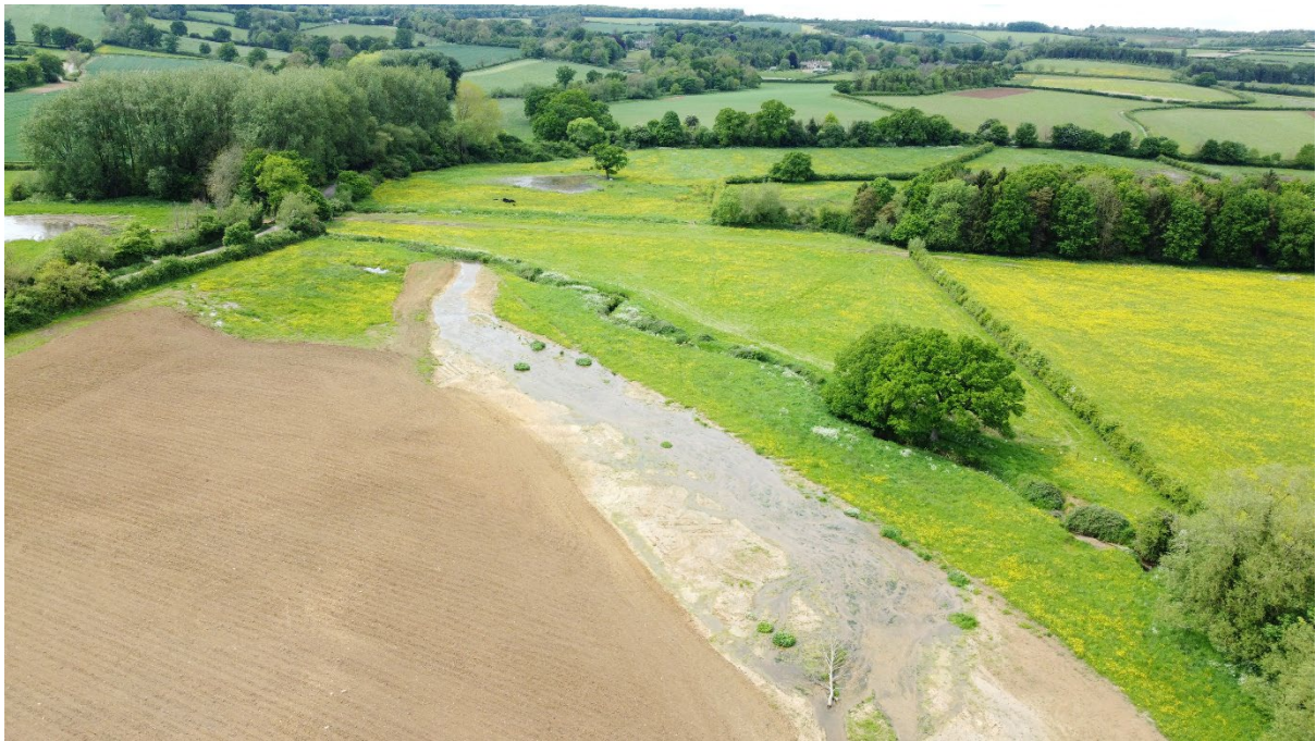
Cornwell Estate River Restoration: Middle section involving partial excavation of channels and removing topsoil. Drone footage [Wild Oxfordshire]
